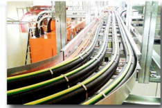
LT/HT Cable Laying
